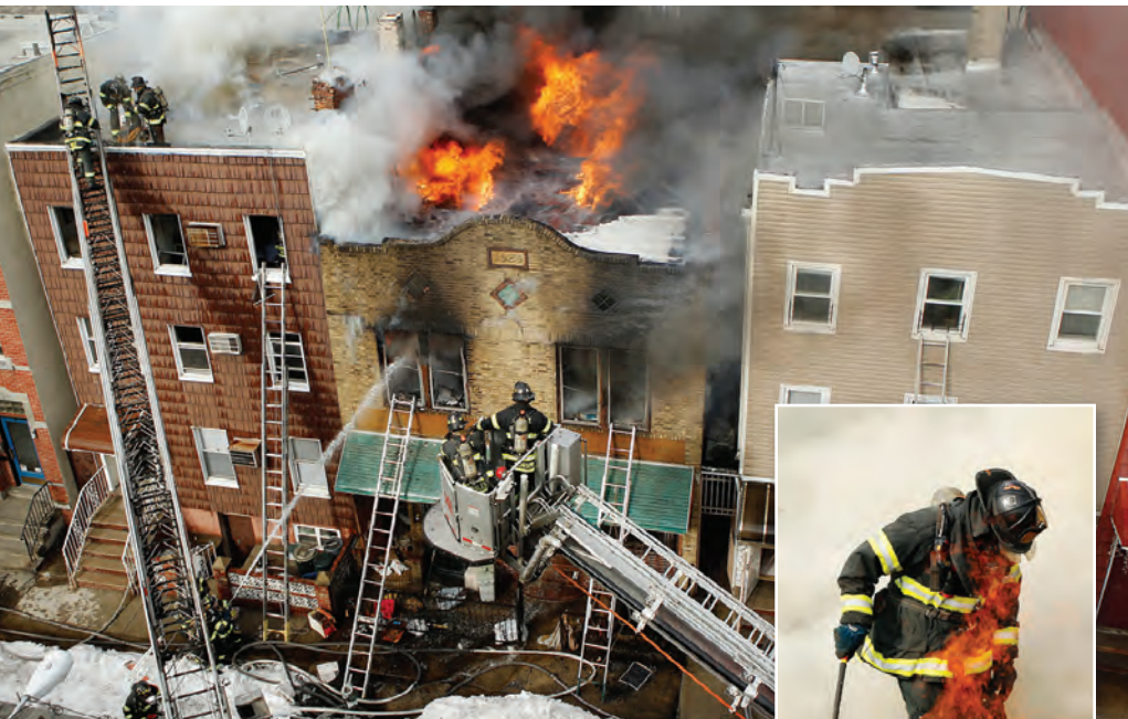
Firefighters from the Fire Department of New York work to extinguish a major fire in Brooklyn on Feb. 7. The fire consumed a two story building and part of a neighboring building.
