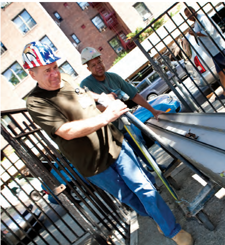
Laborers Giuseppe Dire, left, and Fredrick Colman move steel beams.
